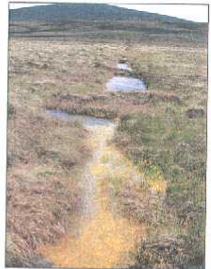
Small peat dams blocking drainage channel in Mountain Blanket Bog, Wicklow Mountain National Park and SAC.
